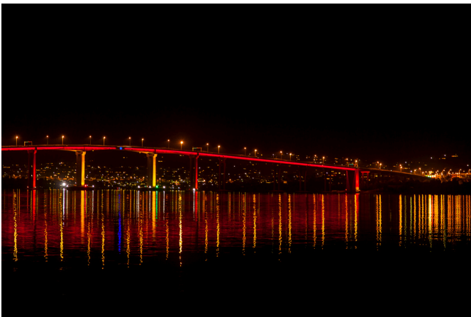
Tasman Bridge, TAS
