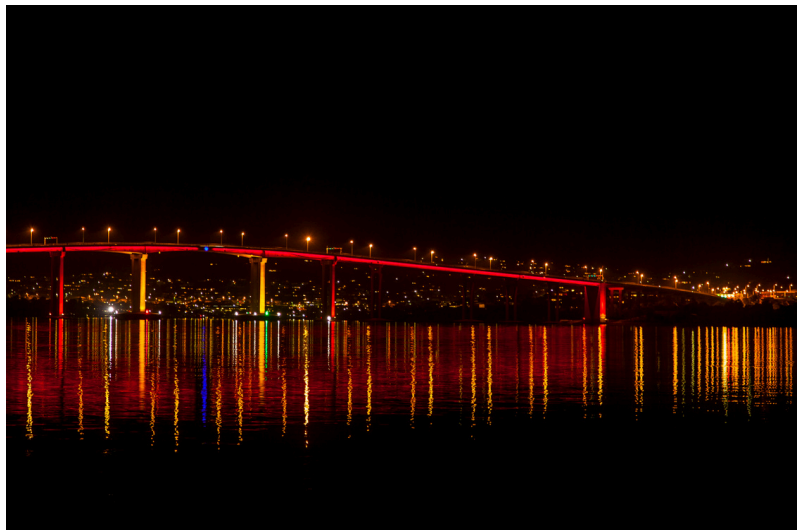
Tasman Bridge, TAS
